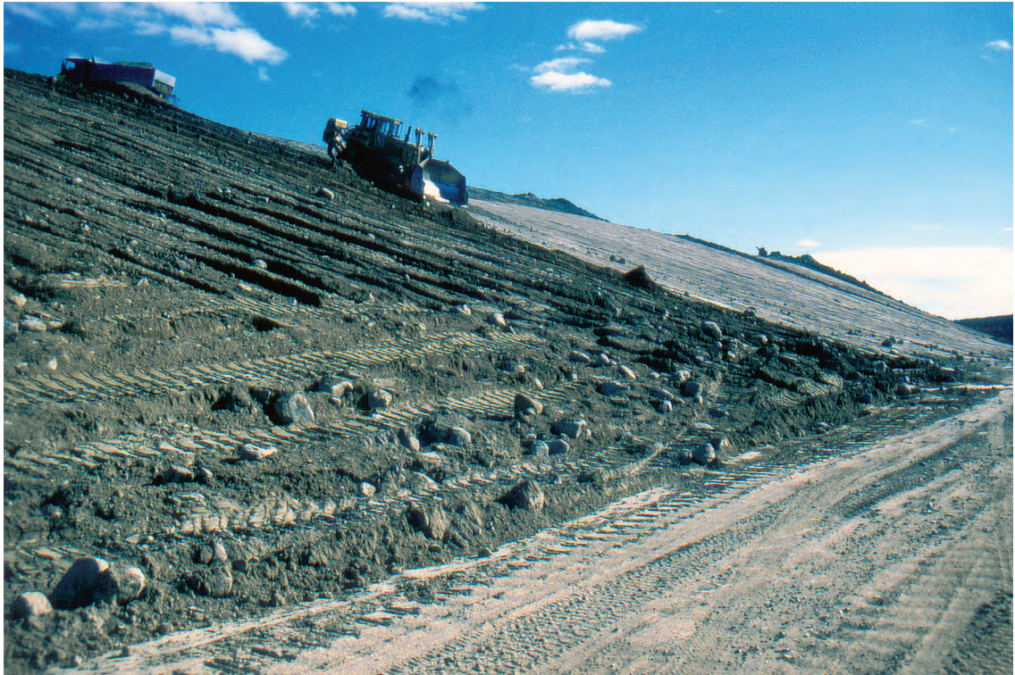
Illustration: Construction of soil cover at the Aitik mine.
