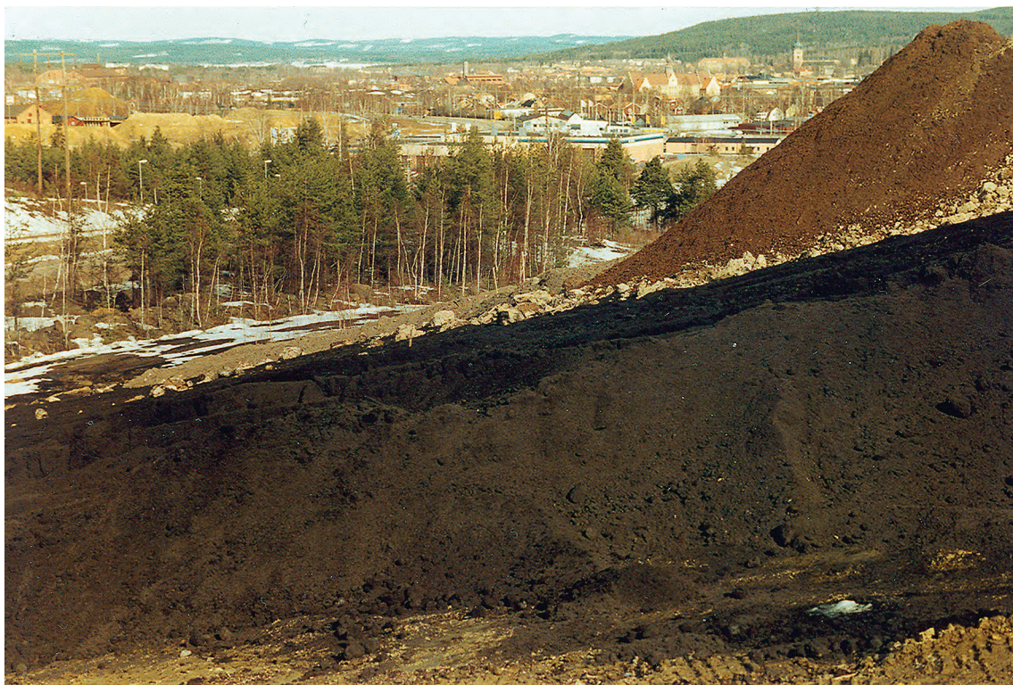
Illustration: Cover construction of fly ash and paper mill sludge at Ingarv impoundment, Falun.
