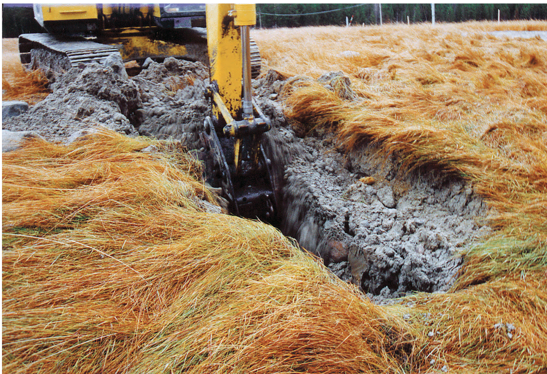
Illustration: Digging exercise in the protective till cover at impoundment 1, Kristineberg.
