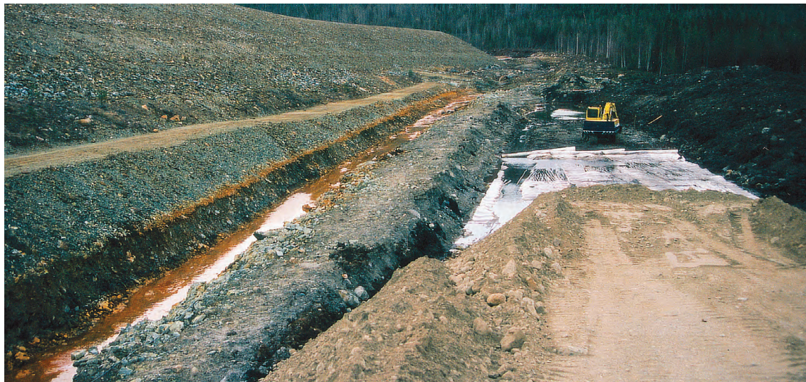
Illustration: Construction work – reinforcement of the dam at impoundment 4 in Kristineberg.
