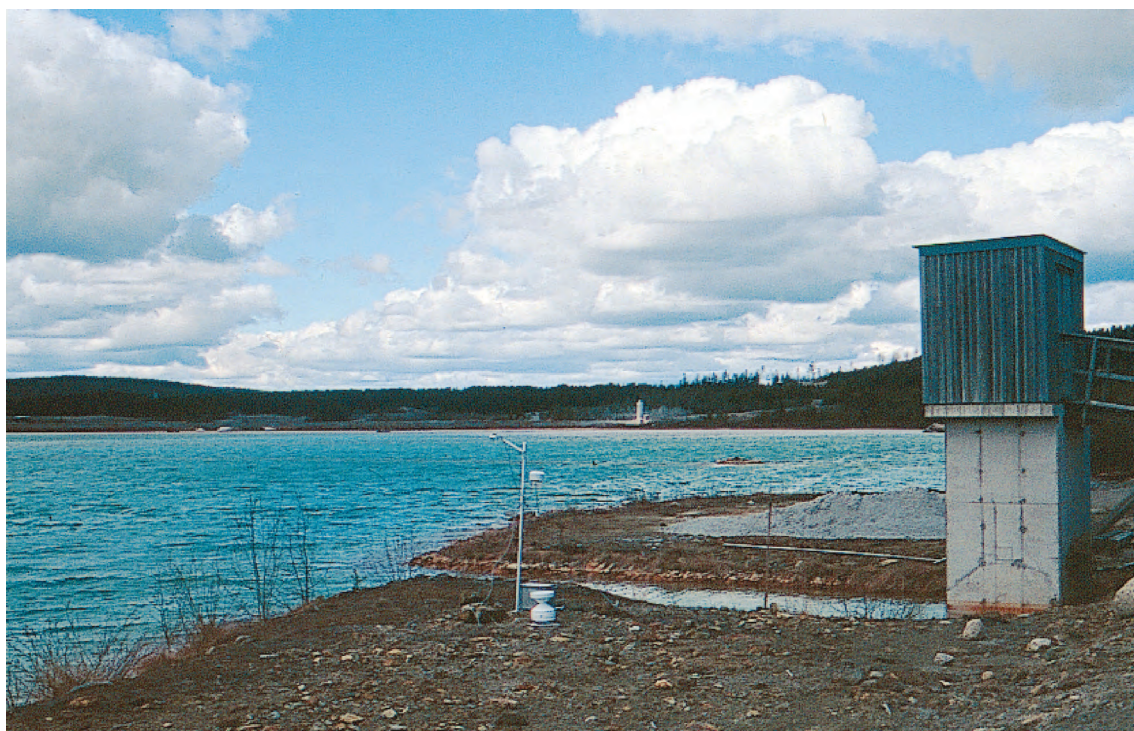
Illustration: Water covered tailings and spillway at impoundment 4, Kristineberg.
