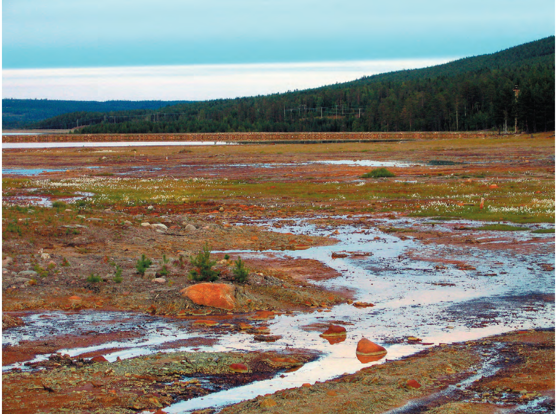
Illustration: Single-layer soil cover with high phreatic surface at impoundment 2, Kristineberg.
